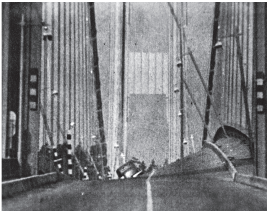
Figure B.67 The Tacoma Narrows Bridge in Washington state in the USA, oscillating before collapsing in 1940, a victim of resonance caused by high winds.
